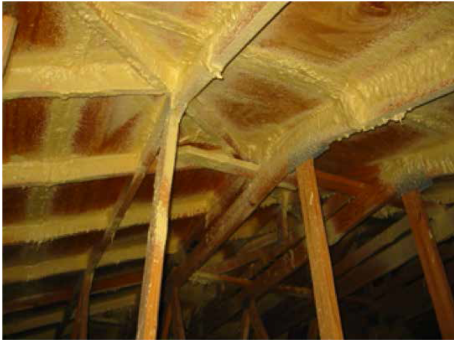
Figure 1. Closed-cell polyurethane foam adhesive applied to the underside of the roof sheathing at the joints between the sheathing panels and along all intersections between roof sheathing and all roof framing members.
